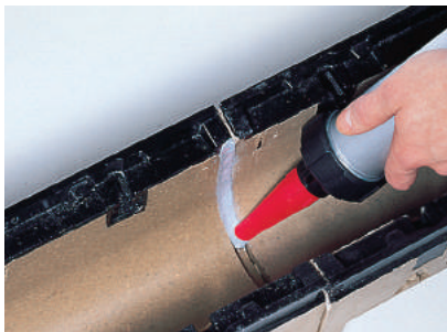
Sealant applied with caulk gun
