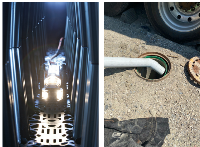
4" pipe with 45° elbow to guide push camera
